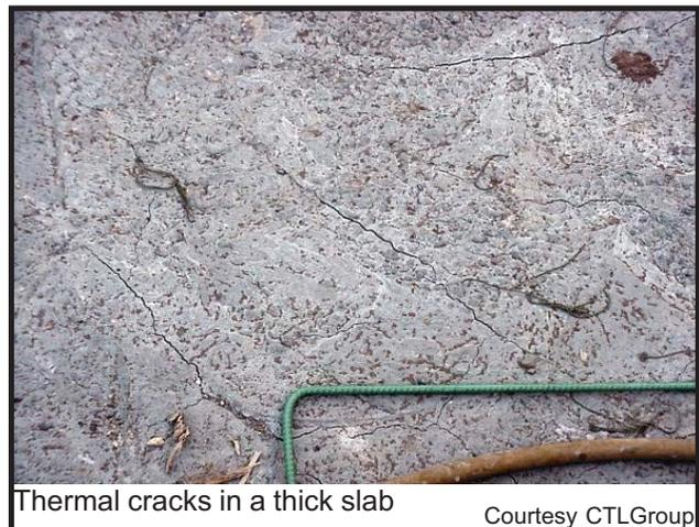
Thermal cracks in a thick slab
